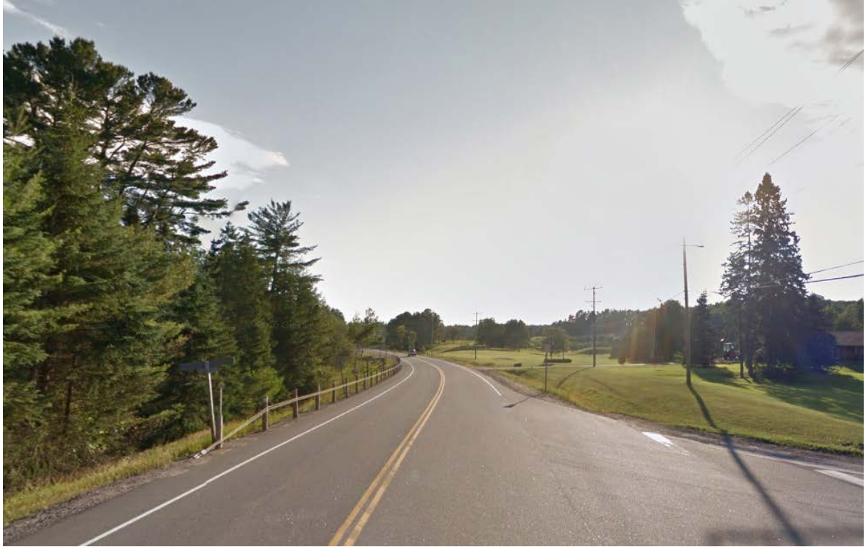
Looking west along Muskoka Road 117 from Muskoka Road 46
