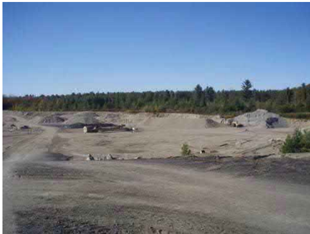
Photo 45. Active operations on existing licenced quarry (October 10, 2011).
