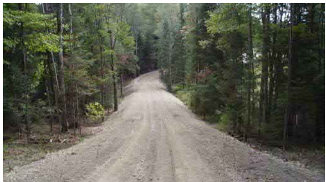
Photo 48. Road constructed and upgraded to access Sage Creek (September 16, 2012).
