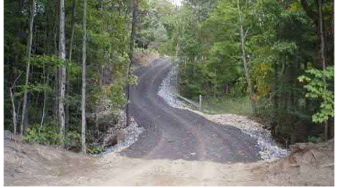
Photo 50. Road constructed and upgraded to access Sage Creek (September 16, 2012).
