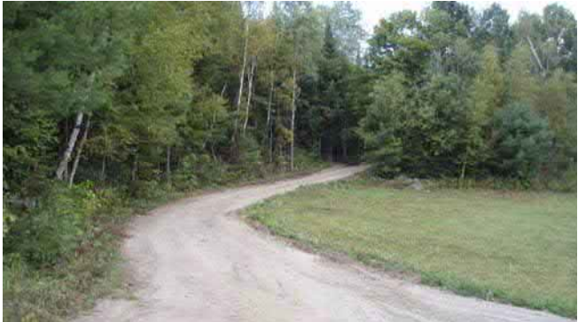
Photo 51. Road constructed and upgraded to access Sage Creek (September 16, 2012).
